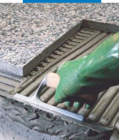
External installation of relief terrazzo "graniglie" tiles
