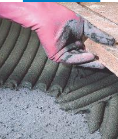
Installation of hand made terracotta on an uneven substrate
