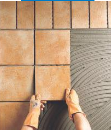
External installation of klinker tiles
