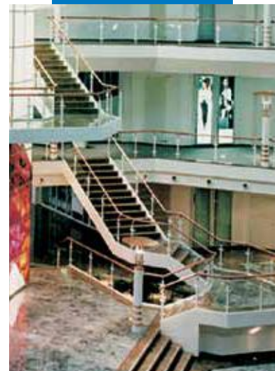
An example of an installation of ceramic or marble on a metal structure (stairs)
