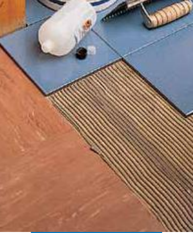
Laying on an old PVC floor
